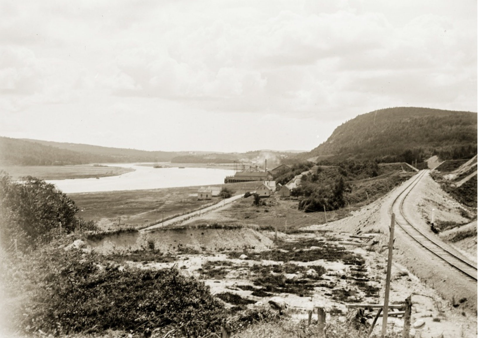
Above: Of the railroad photos, this may be the furthest North in the collection. We are looking at Mount Waldo from Frankfort and the camera is pointed nearly due South. The line is very freshly graded and one can see the level of cutting and the amount of earth that had to be moved to make the railroad grade. Without a documented date it is impossible to be certain but this looks to your editor like late 1905, possibly before the line was actually put into service. PMM LB2015.12.182
