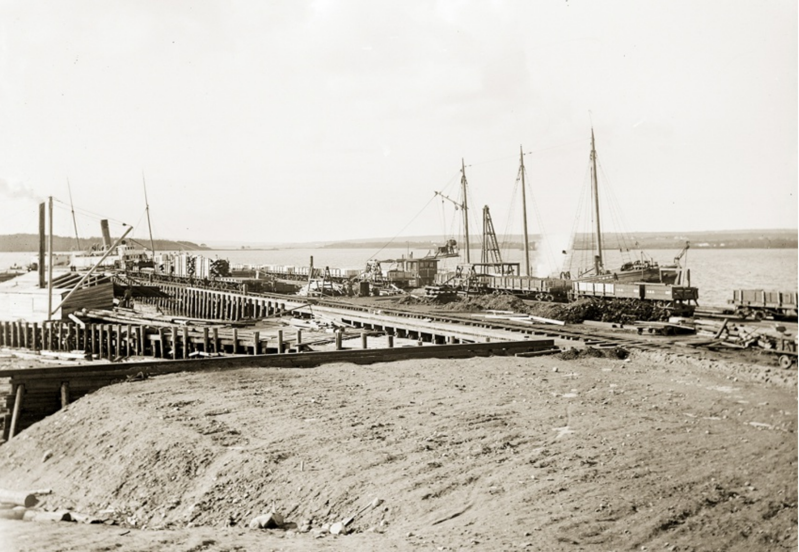
Above: In what is believed to be the earliest photo in this series of Cape Jellison dock images we can see N.M.S. stenciled dump carts on the far track. Note the piles of fill sitting next to the furthest track over and the lack of any sort of ground cover in the foreground. These indicate that this is most likely 1905 or 1906. PMM LB2015.12.24
