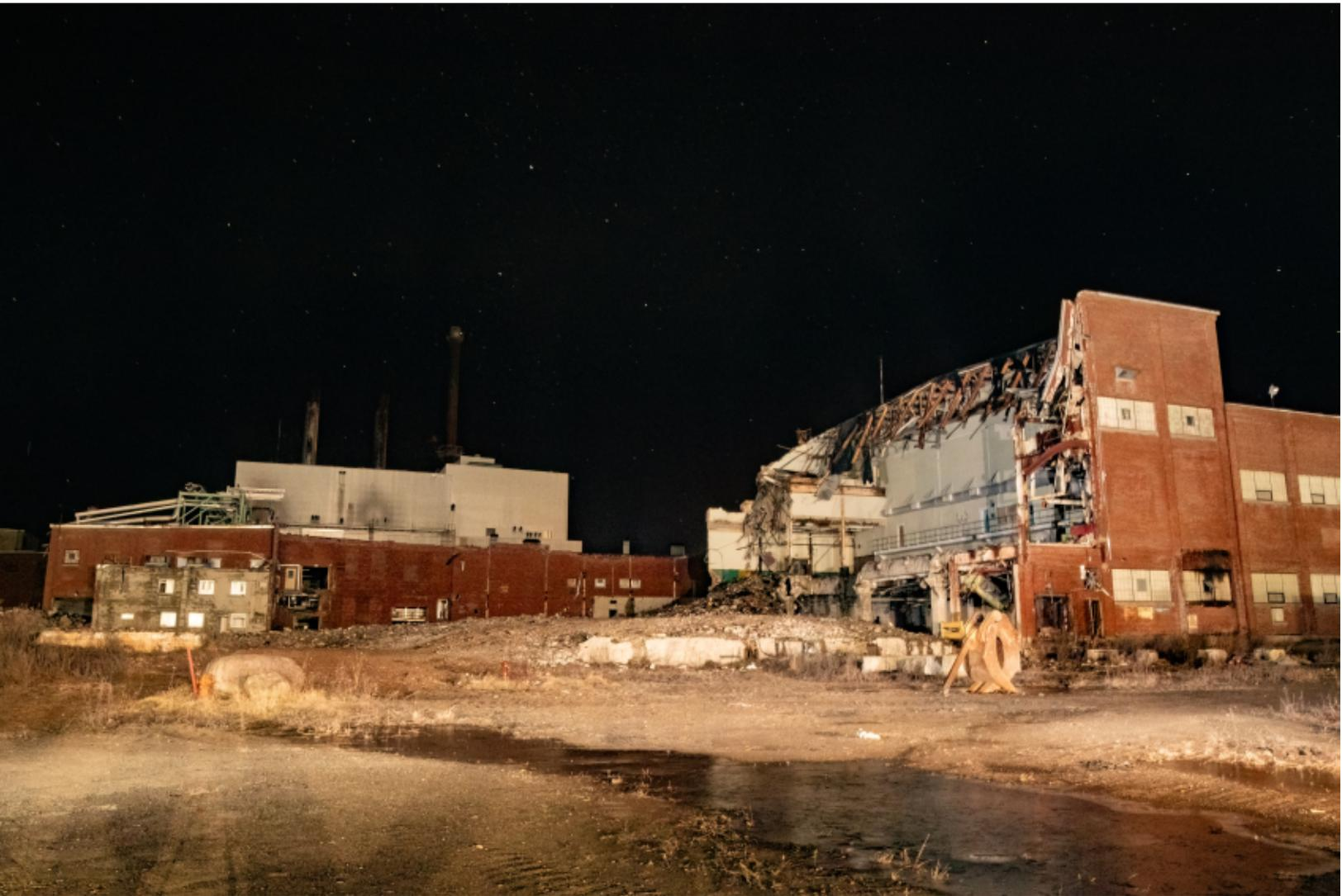
*Above: The pile of rubble is all that remains of the mill building that housed the paper machines. Unable to remove them efficiently, the building was demolished so they could be scrapped.*
