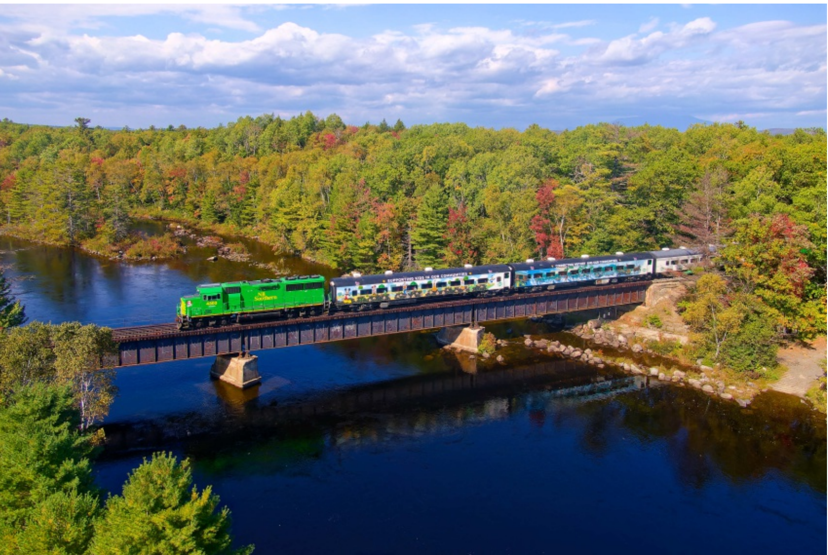
Above: The second run of the day followed the same route, but with the sun out, the Bridge at North Twin really looks spectacular from the air. Photo courtesy of Mike Peverett
