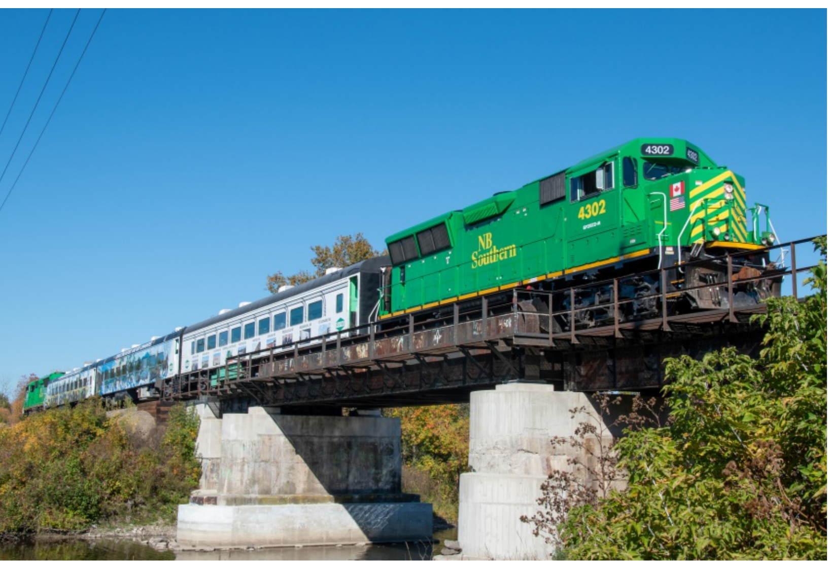
Above: Returning from the first run, 4302 and train are rolling across the Presque Isle Stream.
