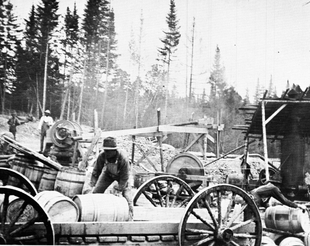
That isn't moonshine in those barrels—This conglomerate of pipes, pulleys and a boiler is not an illicit still operating deep in the Maine woods, but a crusher turning big rocks into little rocks needed to construct the Bangor and Aroostook.
