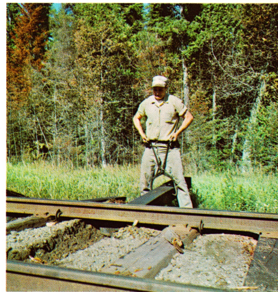
The Job Is Almost Done —With the old tie cut and the ballast scarified, a new creosoted tie is guided into proper position by a member of the tie crew.
