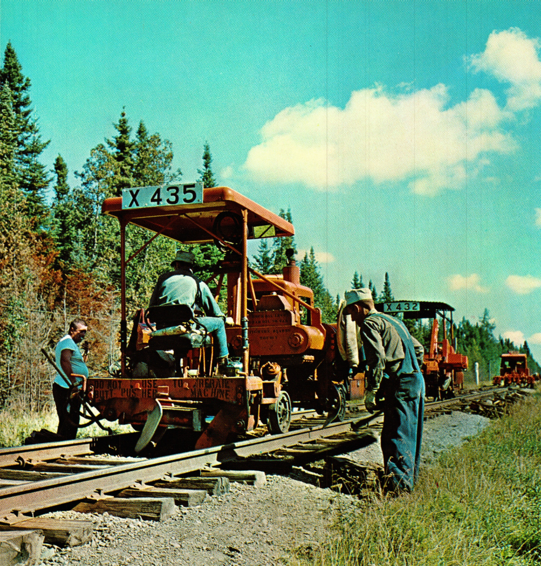
A Machine Makes the Work Load Lighter —This is one of two machines that work as one on the right of way of the Bangor and Aroostook. Its specific job is to cut a tie that is being replaced into three parts, push out the end pieces and lift out the middle piece.
