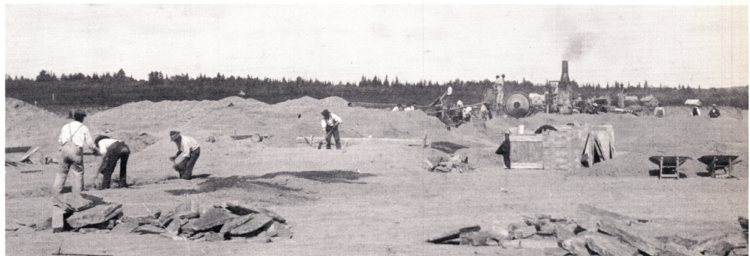
This Was Derby on July 27, 1905— This rare photograph shows the start of construction of the Bangor and Aroostook shops in a hay field not far from Milo. In the background a donkey engine drives foundation piling.
