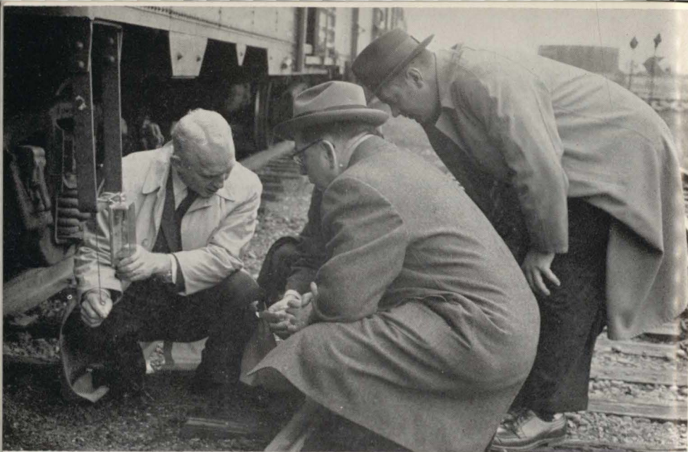
Trainmaster Frank Larlee attaches Impact-O-Graph to measure impacts to paper car at East Millinocket as Traffic Manager Frank Keenan, Great Northern Paper Company, center, and Trainmaster L. S. Milton watch. The Impact-O-Graph is a training instrument for train crews in careful handling of paper.
