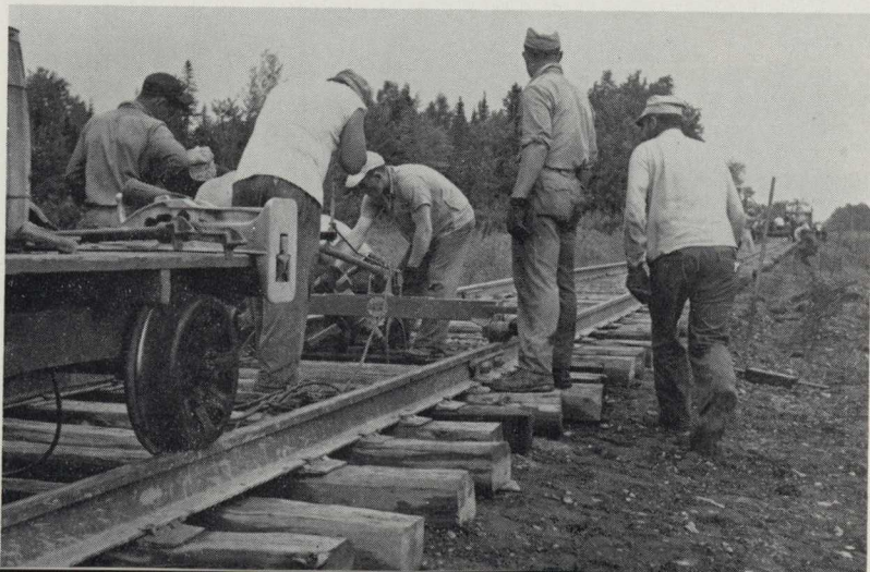
Using assembly line techniques, above, Leo Levesque's crew follows behind plow removing defective ties, and straightening tie plates before ballast train comes by. Below, tie crew uses mechanical tie nipper to hold new tie in place for spiking.
