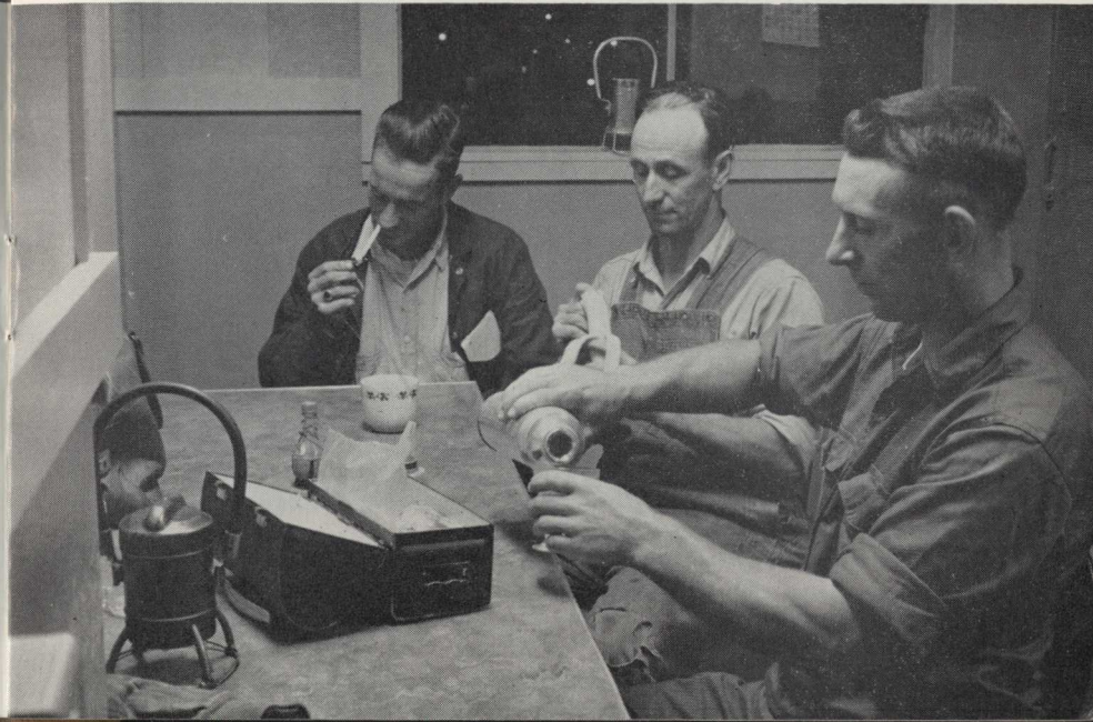
Second floor has lockers, lunch table and desk for train crews. Below, Leroy Bubar, left, E. A. Parks and Carroll Hersey, of the switcher crew, break for lunch.
