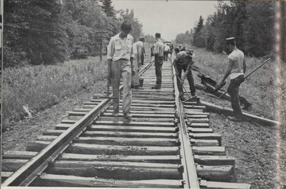
Using assembly line techniques, above, Leo Levesque's crew follows behind plow removing defective ties, and straightening tie plates before ballast train comes by. Below, tie crew uses mechanical tie nipper to hold new tie in place for spiking.
