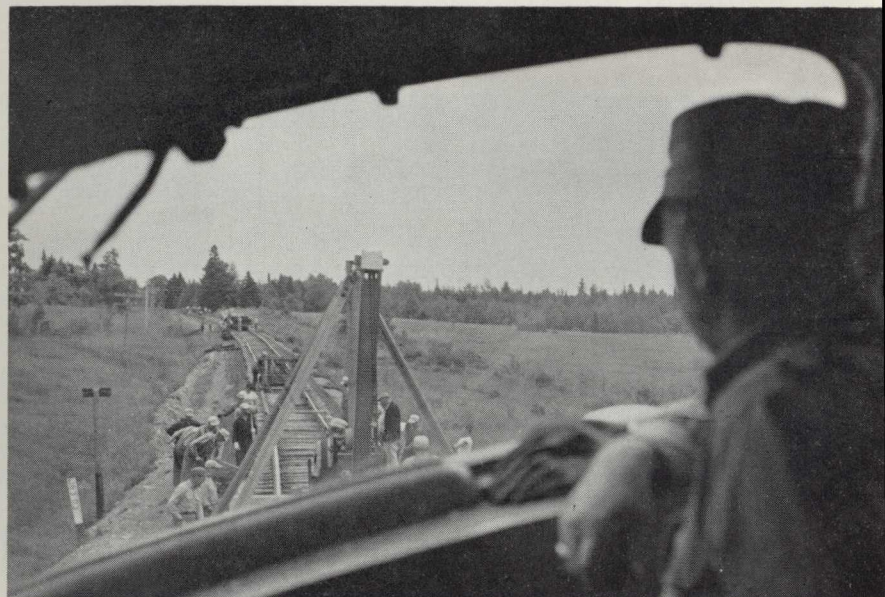
Above, brakeman in diesel cab looks down on plow (similar to sled except for deeper cut). Diesels are coupled to flat car which mounts steel drawbar attached to plow by heavy wire cable. Below, a low angle photograph of sled gives worm's eye view of operating function.
