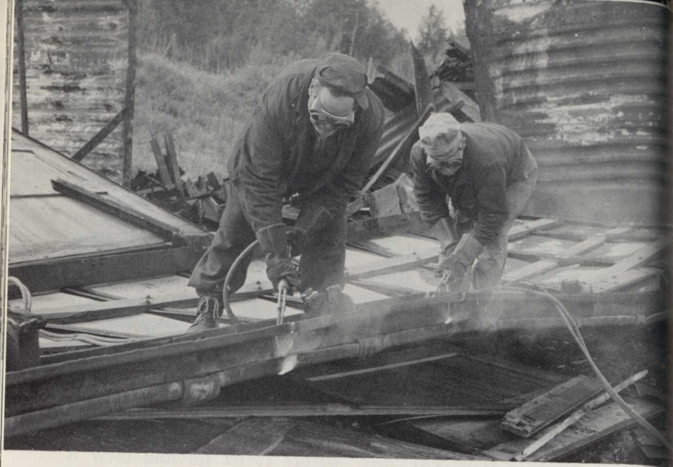
Acetylene Cutters E. L. Whittaker, left, and E. H. King, illustrate the proper attire for the operation. Note tied-down trouser cuffs to prevent hot metal from getting in shoes. Dark safety goggles, of course, are a must for this operation.
