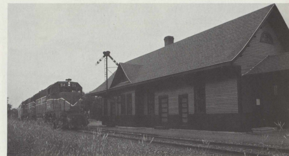
The restoration of BAR's historic Oakfield station by the Oakfield Historical Society and its acceptance by the National Register of Historic Places has to rank as a monument to human persistence in the face of obstacles. The restored structure will be a museum for the Society and is expected to open in time for BAR's Centennial celebration. The Houlton Local, right, highballs past the gleaming structure.
