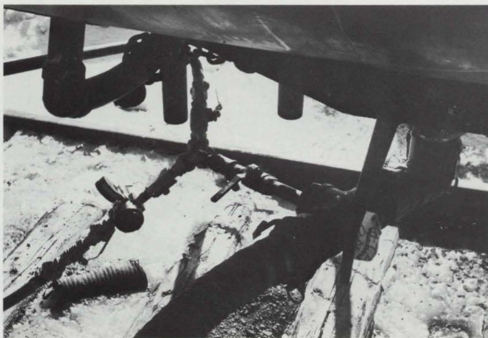
Air is introduced into the tank car to unload latex.
