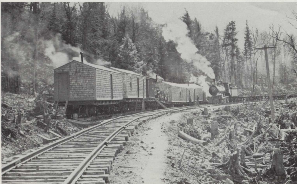
These camp cars housed workers who were building the Fish River Railroad in 1902. BAR Engine No. 19 has steam up and is ready to move an unloaded ballast train. The book contains many historical photographs that have not been published previously.
