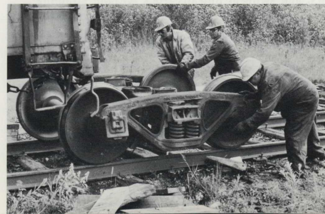
Before the new wheels are installed, Sholler gauges and inspects them.
