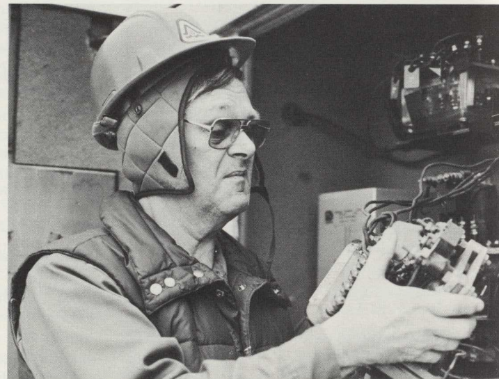
Signalman Fred Bickmore, Presque Isle, holds the traditional relay from a system that will eventually be replaced with state-of-the-art motion sensing crossing protection devices.
