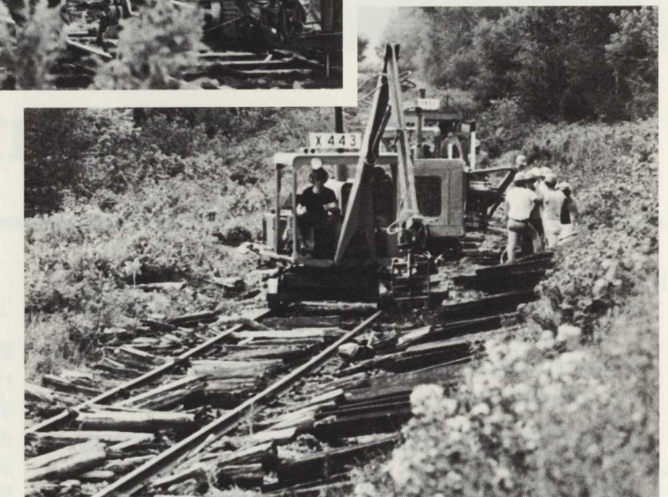
A tie handler removes pieces of old ties prior to insertion of new hardwood ties.
