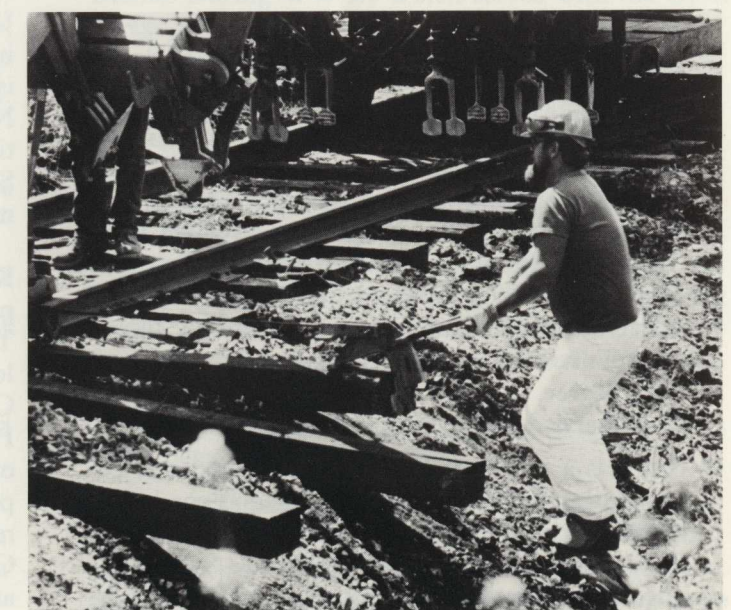
A tie handler removes pieces of old ties prior to insertion of new hardwood ties.
