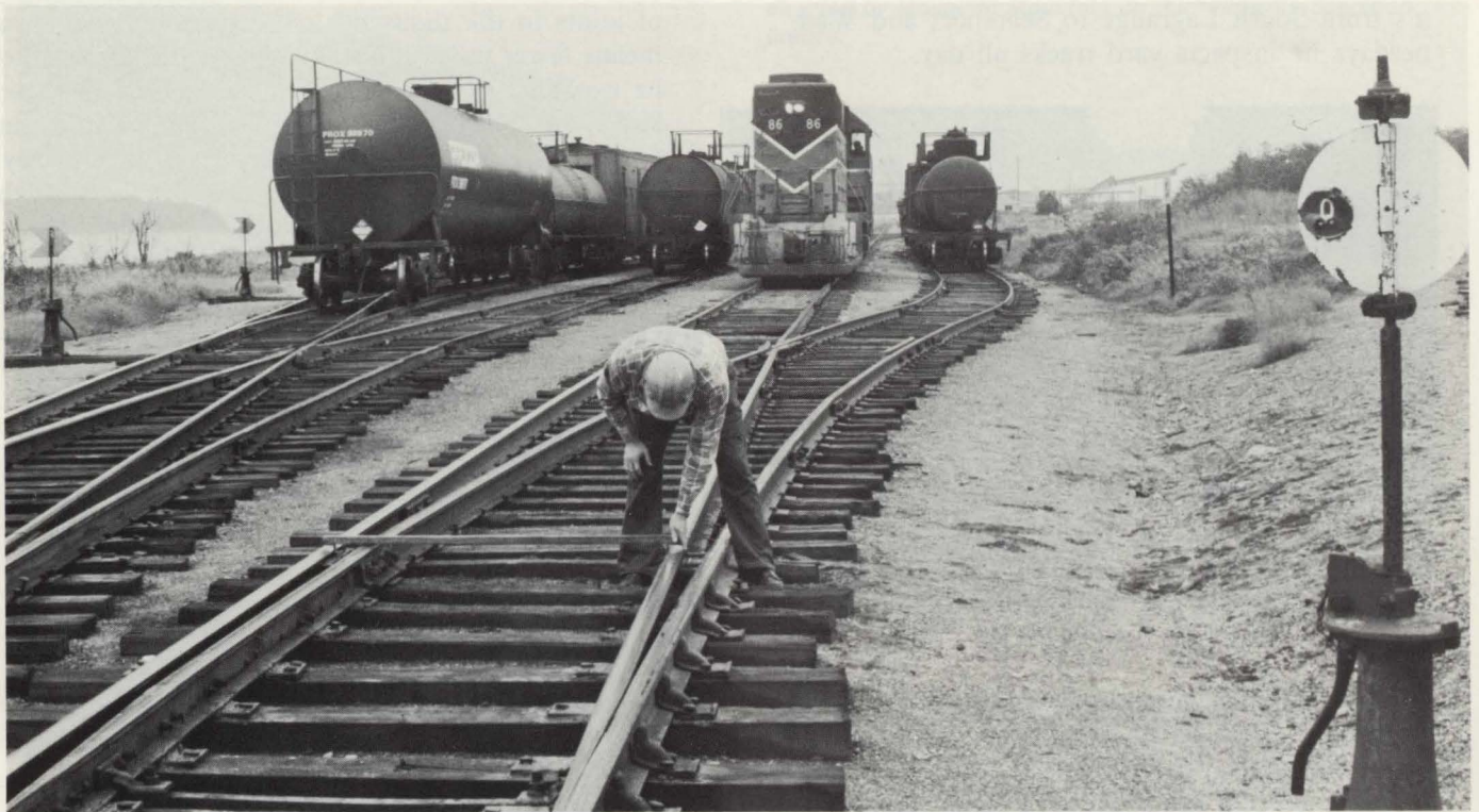
Inspection of yard facilities takes up one day each week of Gordon Cole's patrol schedule. Here he measures the gauge of track in Searsport yard.
