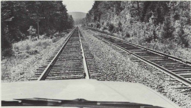
Part of the art of being a successful patrol foreman is to be able to spot defects in the rail from a moving vehicle at about 15 miles an hour. It looks easy but it isn't.
