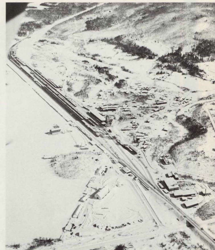
Cripple track facilities at Millinocket Yard, shown in the aerial photograph, will be enlarged and track will be added to service locomotives. Approximately $150,000 will be spent in improvements at Millinocket. The move is expected to generate savings in the half-million dollar range annually on a long-term basis.
