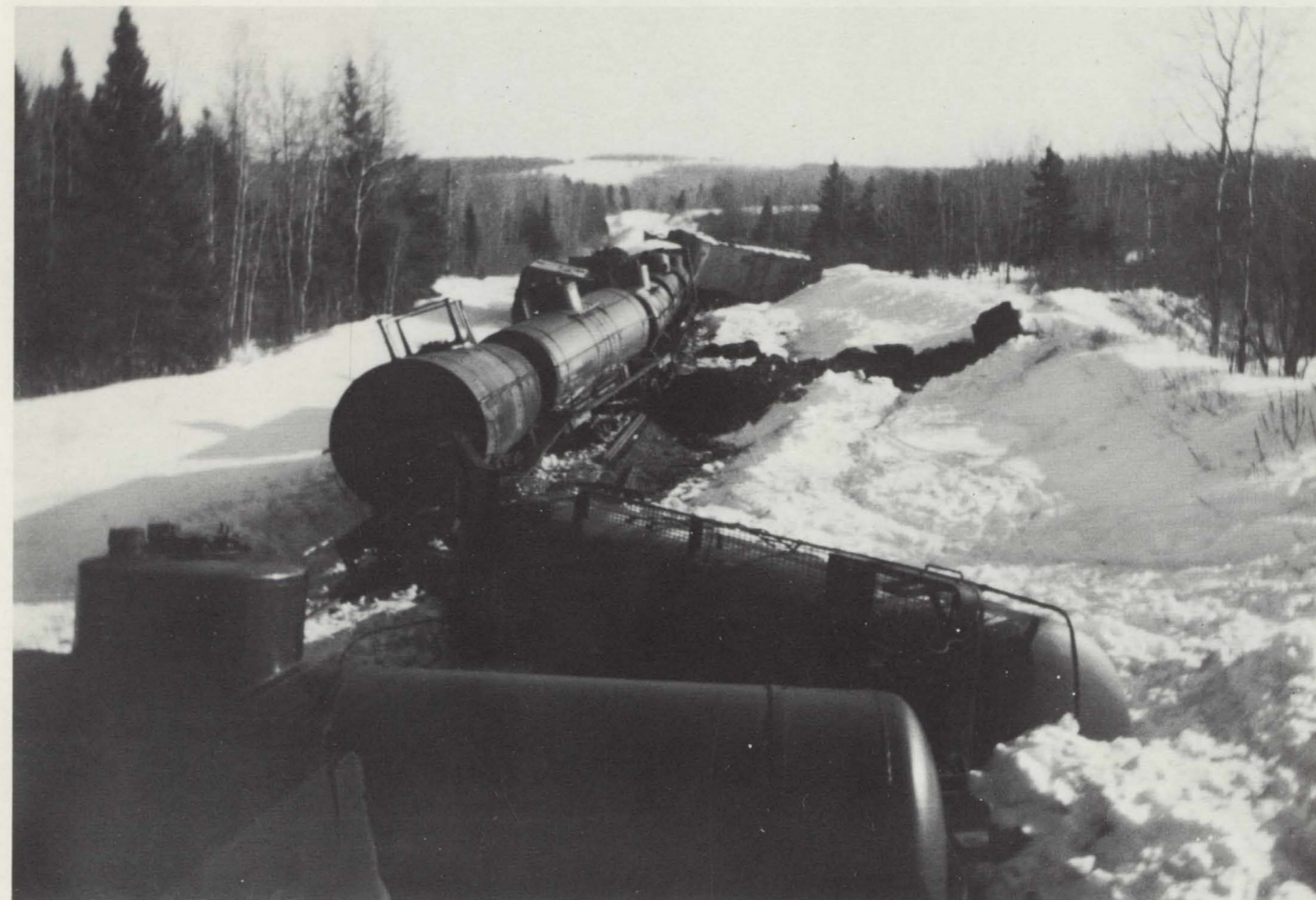
The derailment pictured may not be the typical scene that confronts a wreckmaster, but it probably doesn't miss by much (photo courtesy of L. Marks). John Willinski has been wreckmaster for the Bangor and Aroostook for more than 20 years and, while he doesn't look forward to chaos like this, he's pretty good at picking them up.
