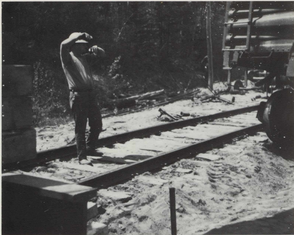
Willinski signals a crane operator dropping a boxcar onto a set of trucks at the scene of a fender-bender type derailment.
