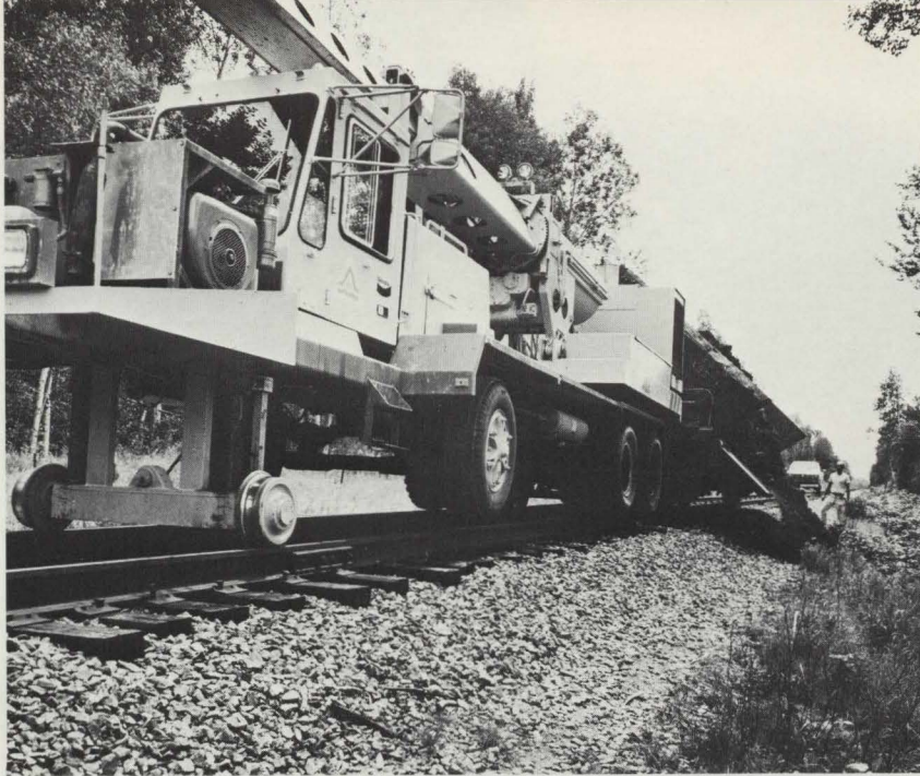
The unit carries its own air compressor for braking and the work equipment includes a side-dump car to dispose of ditching material.
