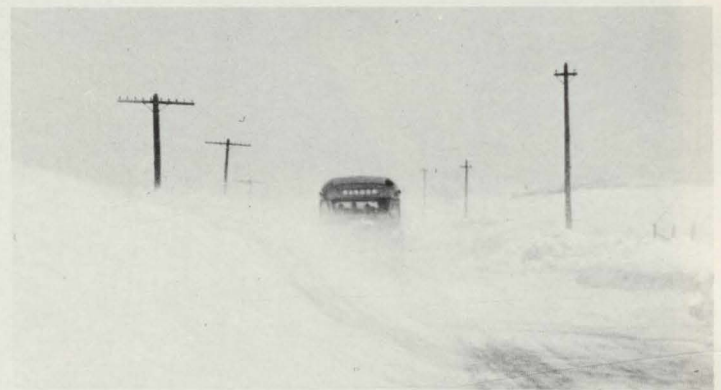
Like the U. S. Postal Service, the BAR Highway Division was not easily discouraged by blowing snow, sleet or rain as this early photograph, bus 102 on the Caribou Road outside of Van Buren, shows. Drifts of snow reach halfway up the telephone poles and nearly to the tops of the bus's windows.
