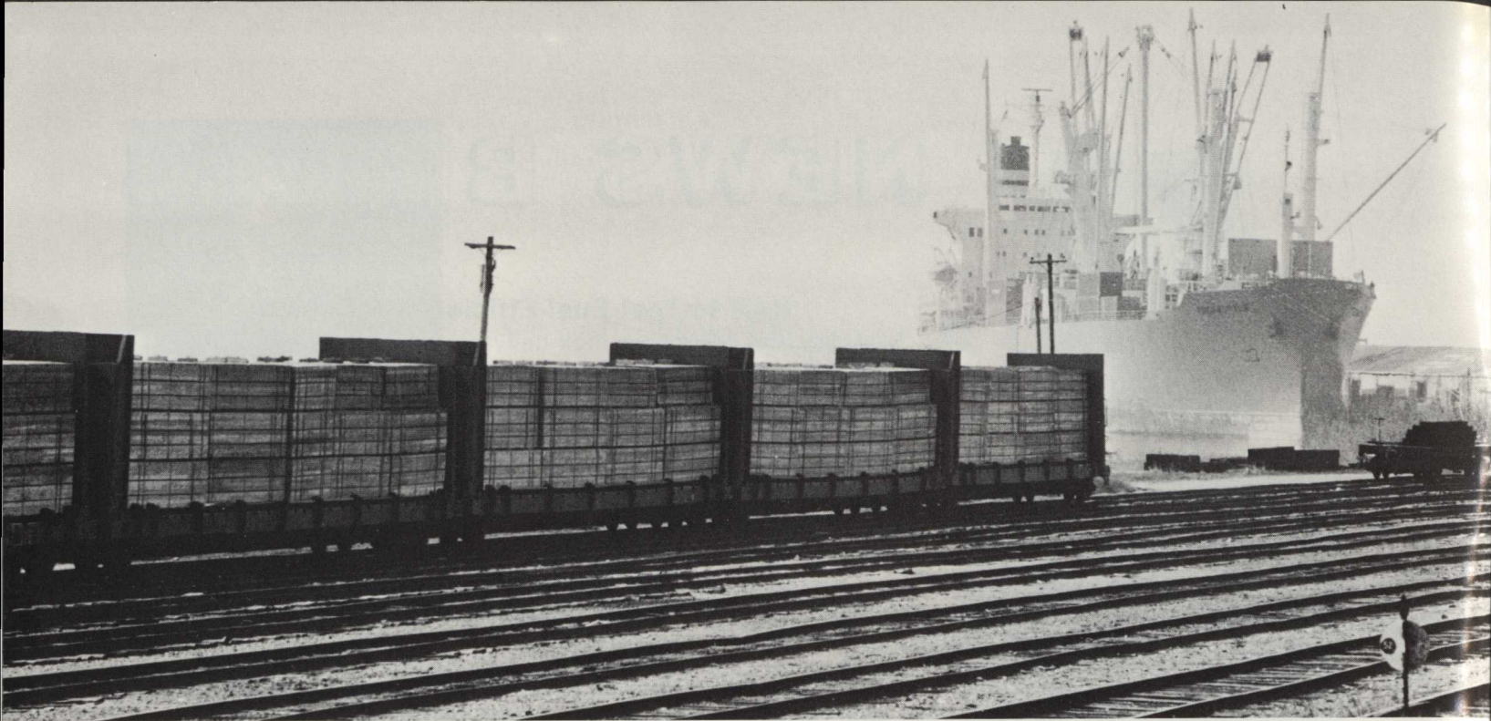
Carloads of lumber sawed by International Paper's Marsardis Mill awaits loading aboard the MEMBERSHIP at Searsport in May. The 3.9 million board feet of lumber was exported by Boscus International and meant 90 carloads of traffic for the railroad.
