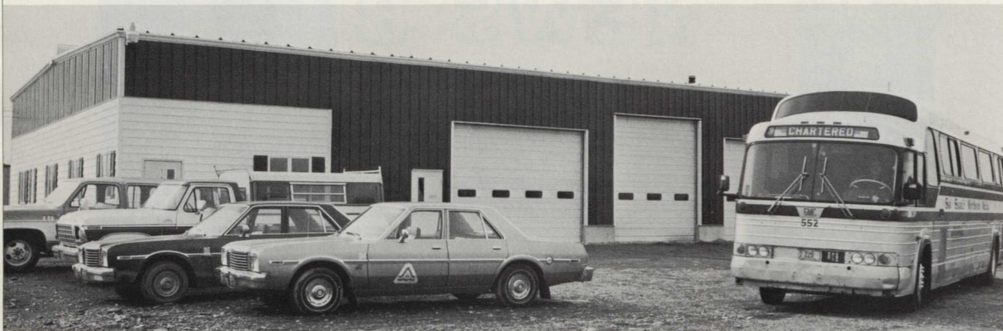
The Bangor and Aroostook's highway division moved into a new maintenance facility in January. The new $200,000 structure houses offices for Manager S.F. Corey and staff as well as quarters for drivers and a modern maintenance shop. It's the first time in the 44 years the railroad has operated buses that administration and maintenance have been under the same roof.
