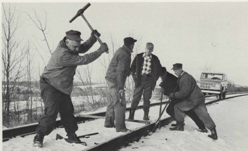
Roadmaster Albert Snow stops to check the progress of Fireman Elden Wilcox and his crew — Sterling Gamblin, Eddie Plourde and Ed Wing — who are shimming track on the Limestone Branch.
