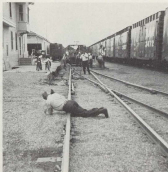
Cleaves made the photograph of his father, Foreman Sandy Cleaves, lining track in Houlton yard during the summer of 1966. Sandy Cleaves made the photograph at left during the hand 'pede days in the late 1920s. Pictured are Foreman William Gilpatrick and Wallace Bolstridge near Buffalo on the Ashland Branch.
