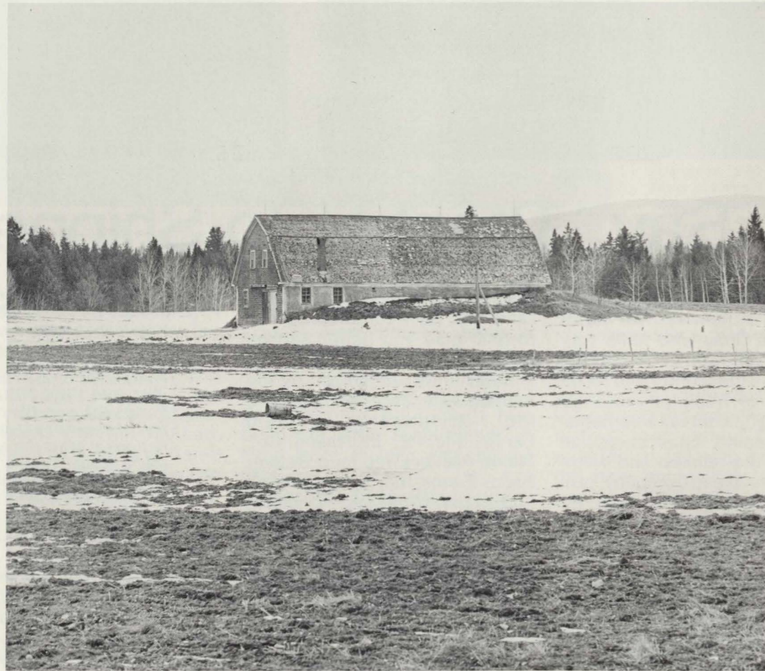
The Aroostook potato house is a storage uniquely adapted to the needs of the northern Maine potato grower. It is typically half-buried in the earth and, because of a series of low-price years in the 60s, increasingly in need of replacement. Higher crop prices promise a surge of rebuilding and the railroad is campaigning to persuade shippers to build their storage on rail so they have a choice in shipping.
