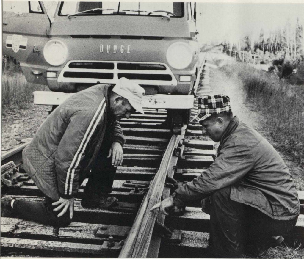
Using a hy-rail truck Track Inspector Ralph Tozier, right, and Trackman Beverly Smith examine a switch point for wear on an early-morning run on the Searsport Branch. The photograph below of a shimming operation on the Van Buren branch was made April 10, 1934 and shows a type of motorcar in use at that time. Note the absence of canopy.
