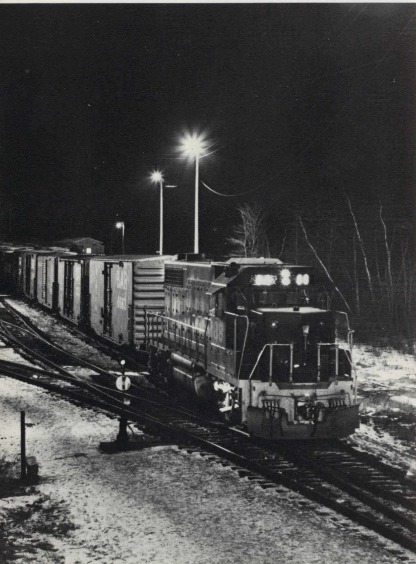
Railroads, long the "disadvantaged" of the transportation industry, have the tools to correct many of the environmental abuses that the public demands be righted. Railroad facilities, like the BAR's Northern Maine Junction facility pictured here, do not interfere with travelers using public facilities. Air pollution from railroad is one-fourth of that of highway carriers and rights-of-way are privately-maintained.
