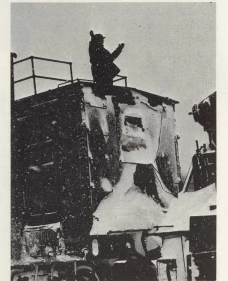
A machine like the Pettibone, being used in snow removal in the top photograph, presents a potential hazard to railroaders working in yards and sidings where such equipment is being used and requires extra care. The foreman below is giving directions on a spreader train clearing one of the railroad's yards. Extended wings on spreaders or plows can assault the incautious trainman or trackman.
