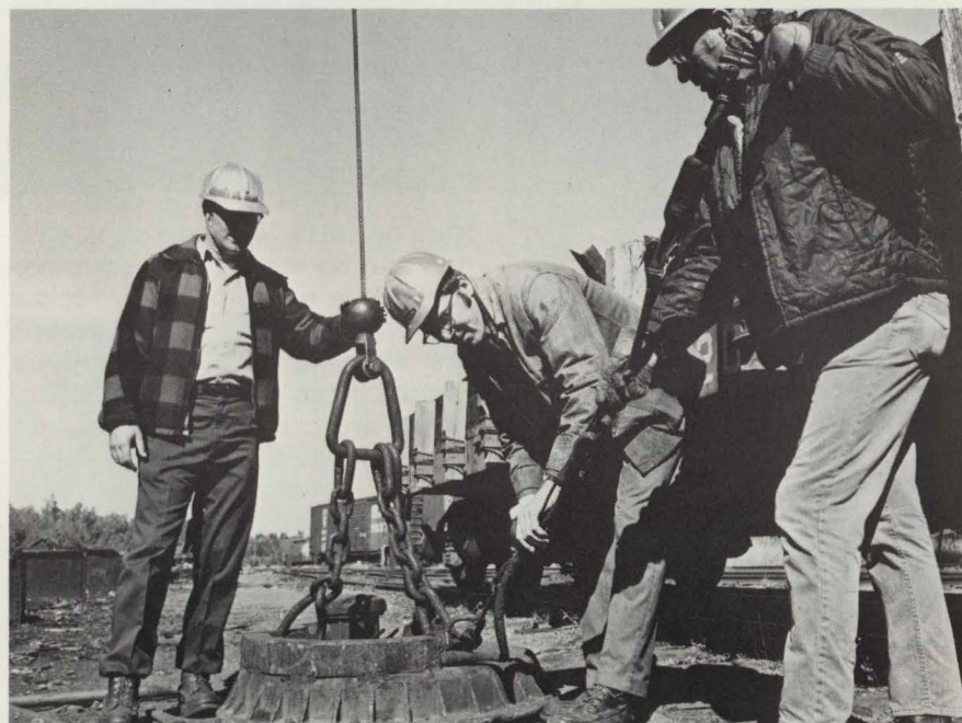
Above, Foreman Alan Hearn, left, watches as Purchases and Stores men Roland Richardson and George Hussey ready the electro-magnet on the department's crane. Hard hats and safety shoes are mandatory for the job.
