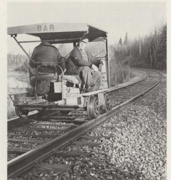
Motocars like this one are being phased out. The section crews formerly spent part of their day just patrolling track. Now, under the maintenance point concept, crews are larger and mostly use trucks equipped with hy-rail attachments.
