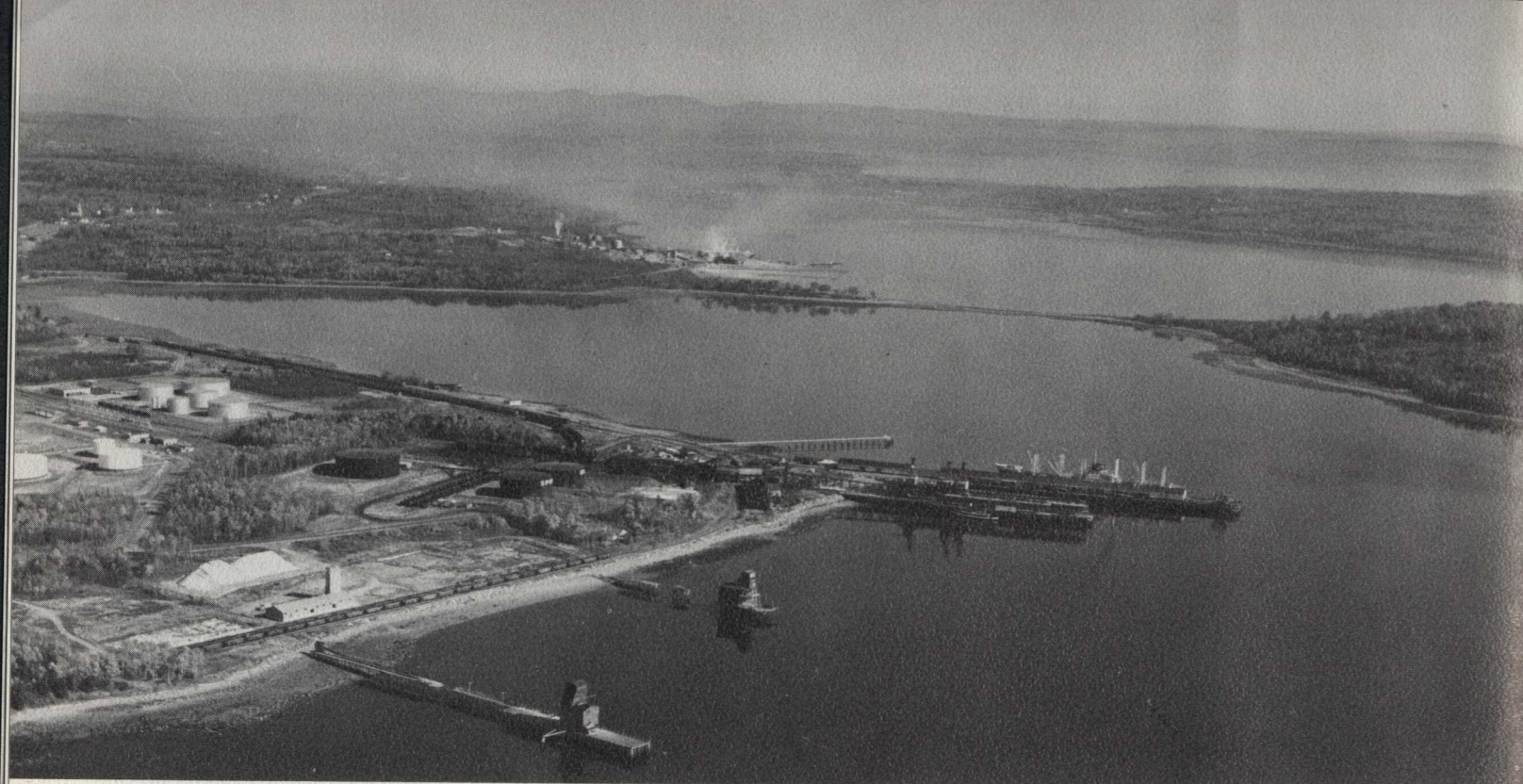
An aerial photograph of Searsport Harbor shows the Bangor and Aroostook's docks and C. H. Sprague facilities in the left foreground. The tip of land at right is a portion of Sears Island and, in the background, the Delta Chemical plant can be seen. Maine Clean Fuels, Inc., has applied to the Maine Environmental Improvement Commission for permission to build a desulfurization plant on Sears Island. The plant would mean between $4 and $6 million a year to the railroad in increased revenue.
