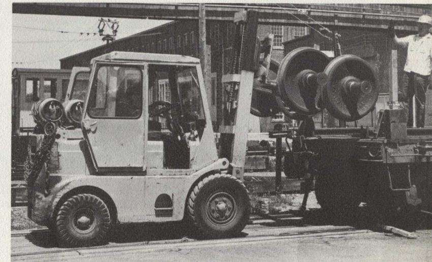
Gone are the days when material at the Stores Department was handled with wheelbarrows and brute strength. The forklift truck and other labor saving devices make easy work of material handling. Above, a forklift loads wheels onto a flatcar for shipment to an outlying mechanical facility.
