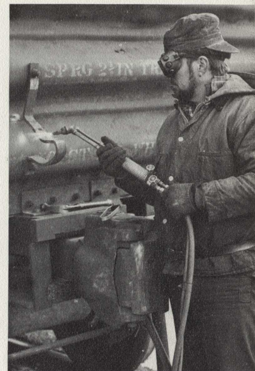
Above, Car Repairer George Hodge heats iron work on a car for straightening. Left, Car Repairer Helper Joseph Vettrano lifts part of a truck for repairs.
