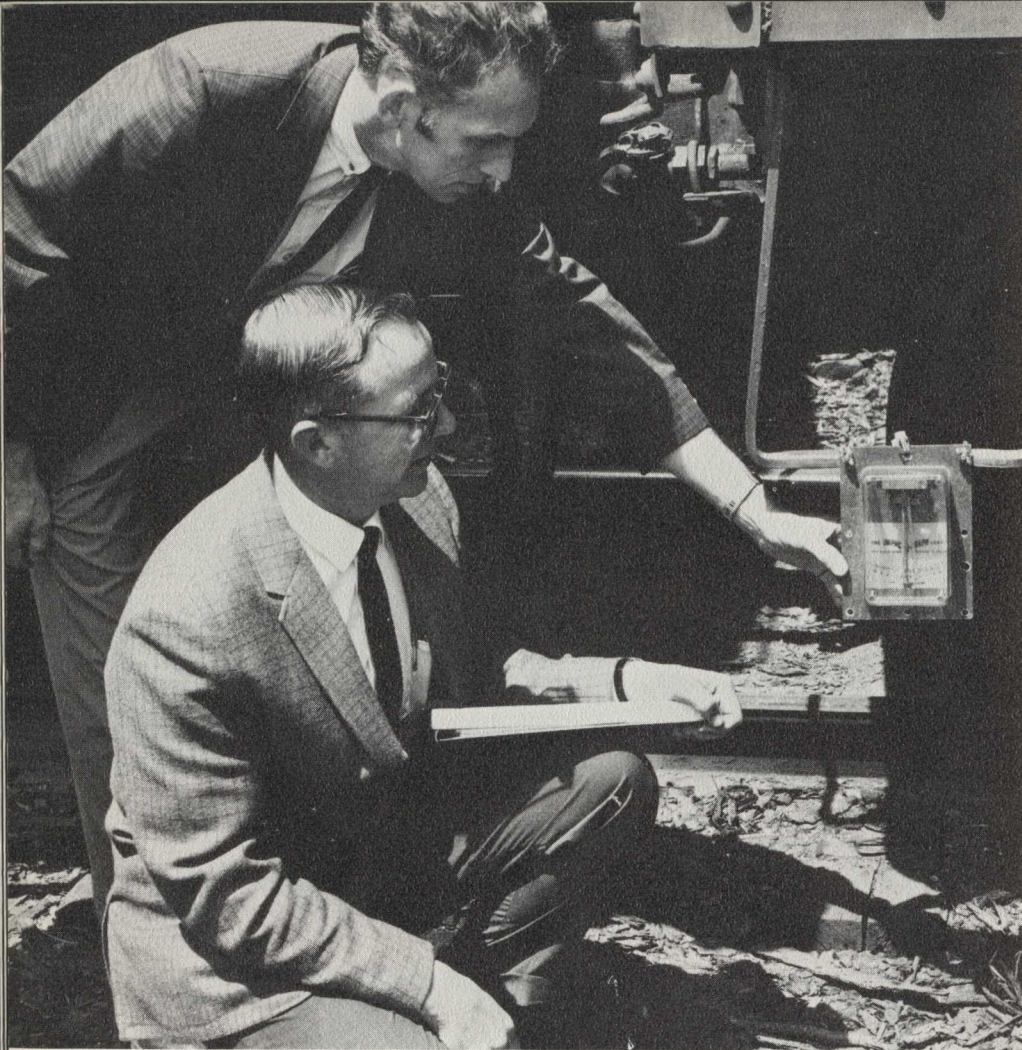
General Yardmaster Irving Foster, Millinocket, (standing) and Damage Prevention Agent George Mossey check a training device which measures impact of coupling during a switching operation at Millinocket yard. Train crews are very much aware of the danger of overspeed impact and the results on newsprint and paper.
