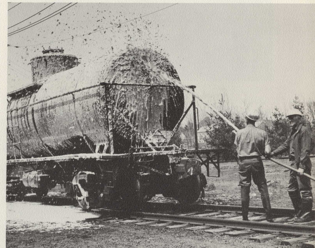
Car Repairer Galen Carey, Derby, and Carpenter Elmer Cunningham direct a stream of foam to cool down a tank car at Derby Shops. In a derailment, foam is used to cover flammable liquids spilled from cars.
