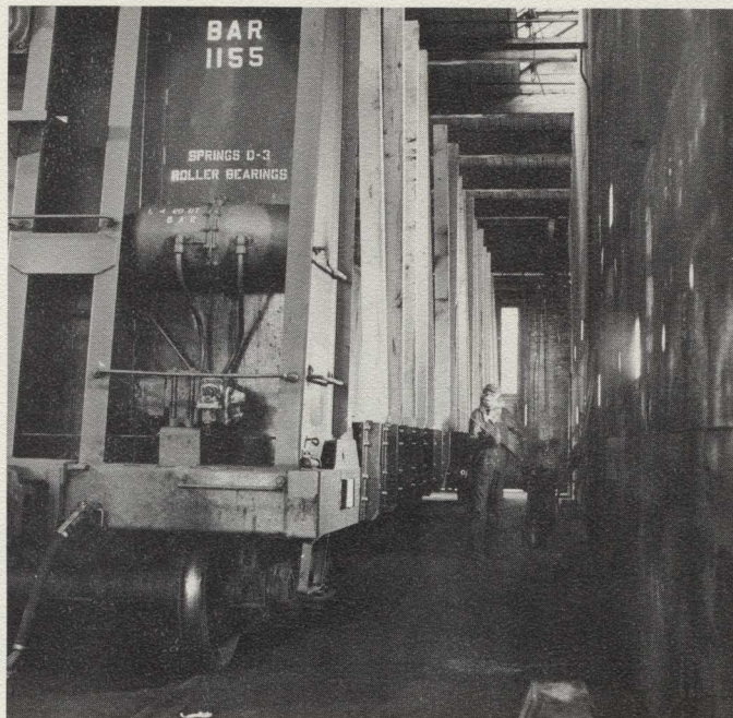
Above, a converted end rack lumber car gets a paint job as the final step in the production line before being placed in lumber service. Below, stake pockets are bolted together before being applied to the car. Some 48 stake pockets are applied.
