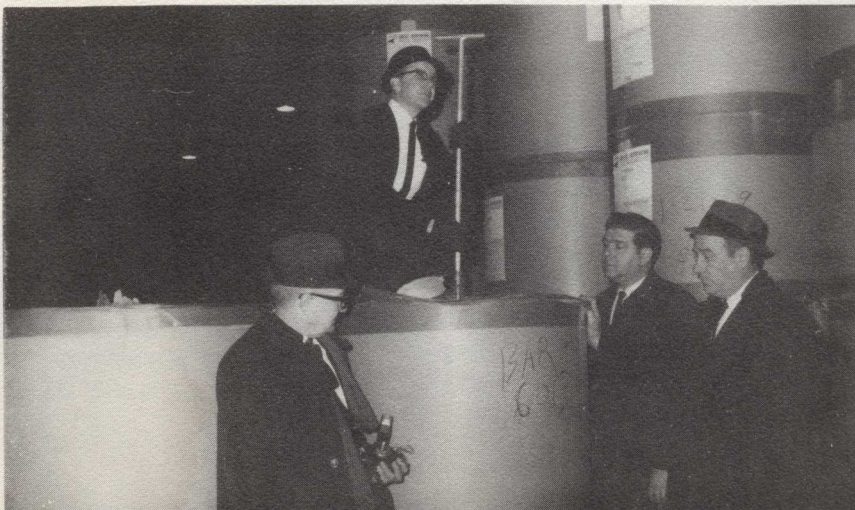
Testing paper cores to determine if the car has been subjected to rough handling are Roland Keefer, AAR; George Mossey, George Stanley, MEC; and Harry Vaughn, B and M. The photograph was made at Star Storage, Inc., in Pittsburgh.
