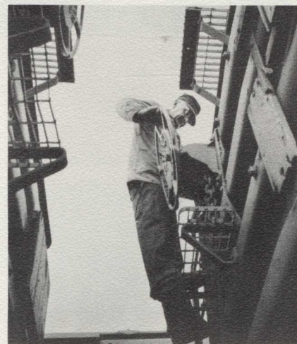
The body must be in the proper position in throwing a switch or the brakemen can lose footing if the handle sticks, then lets go.
