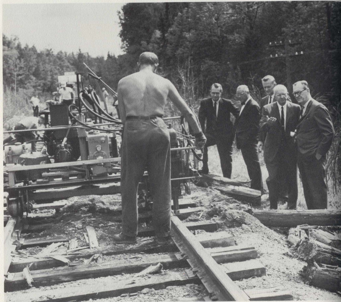
Directors of Bangor Punta Alegre Sugar Corp. watch rail spikes being driven by highly-automated machine during stop in two-day tour of the system.
