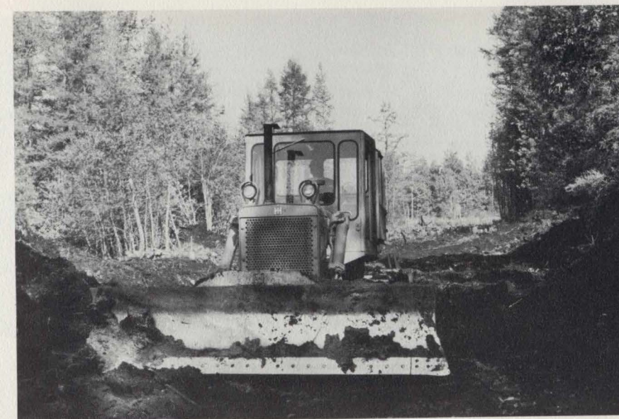
A Bangor and Aroostook bulldozer clears a right of way through a grove of trees for track to Herschel Smith's new potato storage and packing facility in Mars Hill, seen at left during the earlier stages of construction.
