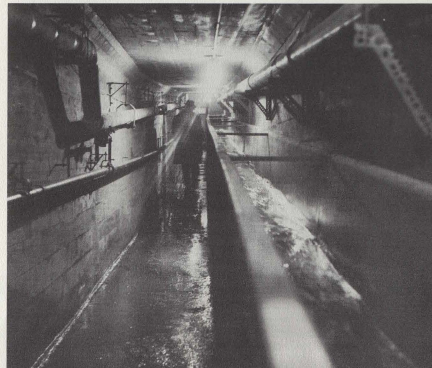
This 140-foot tunnel and flume, deep beneath the Bangor and Aroostook tracks at Washburn, moves potatoes for processing from Washburn Warehouses new potato conditioning warehouse to the Taterstate plant across the tracks, in a flume of water.
