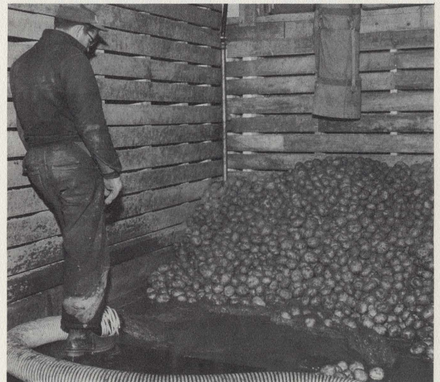
The use of water for fluming potatoes from bins grading and packaging lines is growing in Aroostook County. The installation pictured here is part of a house built by Harold Haines, Presque Isle. Haines plans to build other facilities like this for leasing.
