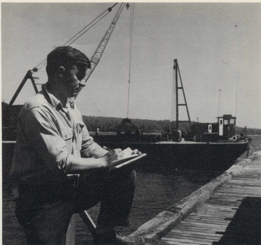
Project engineer O. Dale Anthony meticulously records progress of dredging in his notebook. Great care is taken to assure good safety factor between published depth of berth and actual depth. Framed in warehouse doorway, below, lighter takes a final scoop before moving position.
