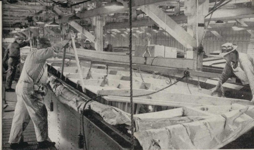
Production line construction speeds new Bangor and Aroostook cars to Northern Maine shippers. A prefabricated roof frame slides on at Pacific Car & Foundry Plant, Renton, Wash.
